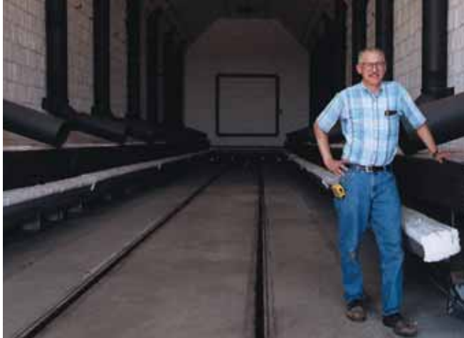
Joe Stitz of Arrow Tank stands in the entrance where rail cars enter the new Arrow Tank heat treating furnace.
